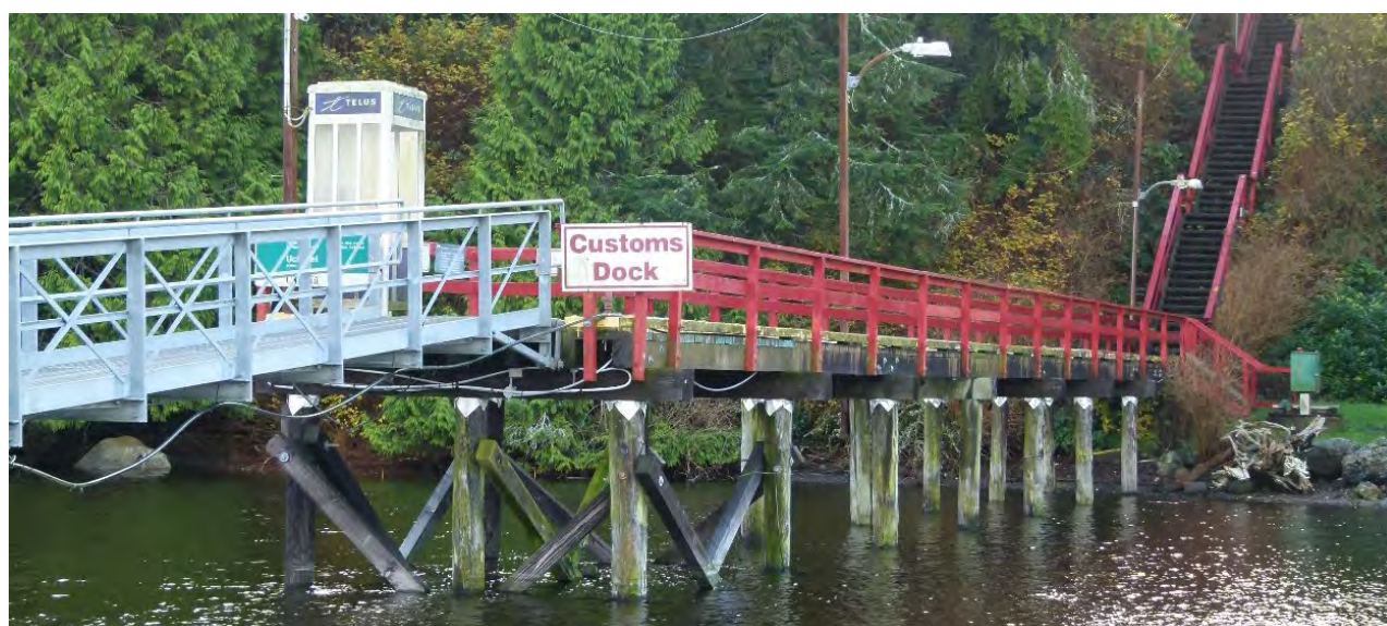
Image 3. 52 Steps Dock - Stair Access
